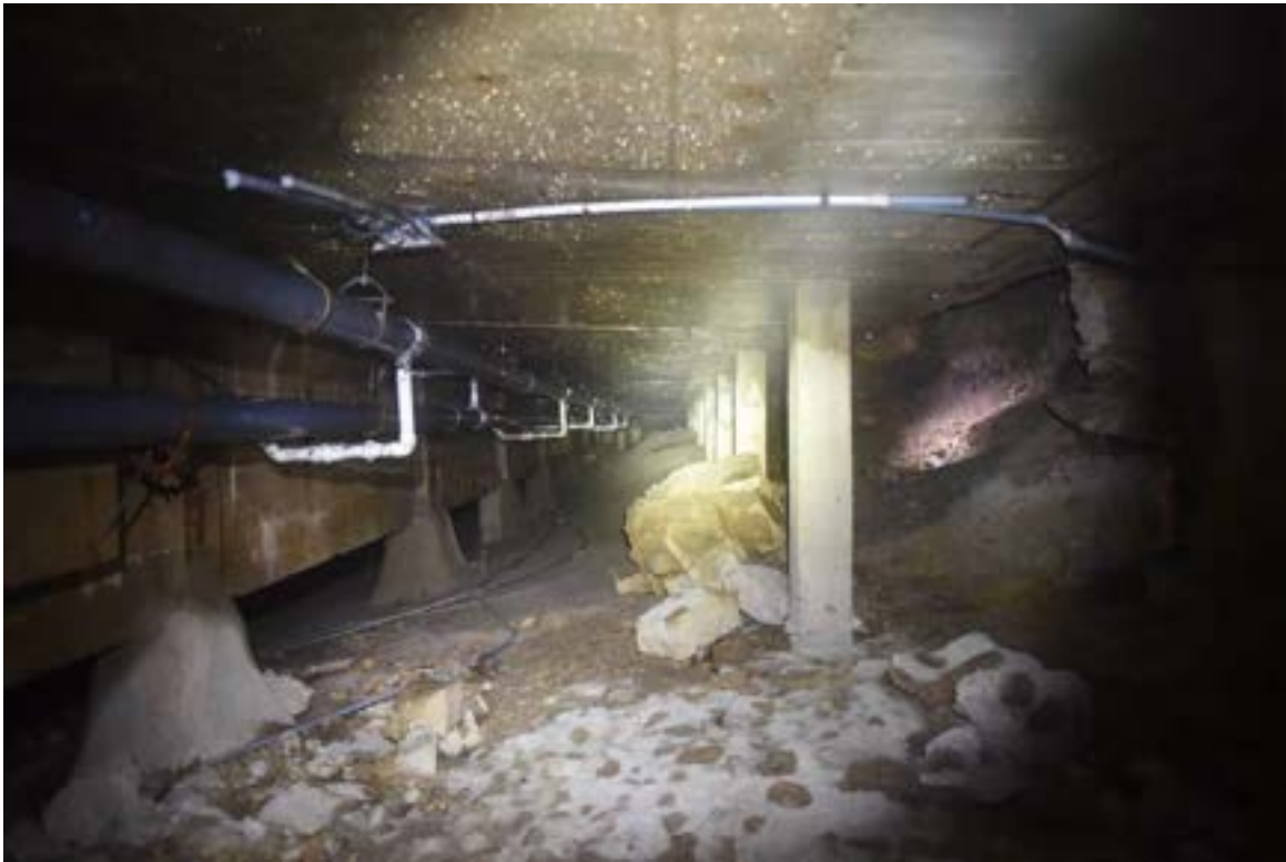
Figure 11. Below the west/northwest side pool deck, looking southwest from the entry point at the box culvert. The pool structure is on the left; rubble of the collapsed stone masonry wall is visible ahead; The retaining wall at the edge of the basin is on the right.
