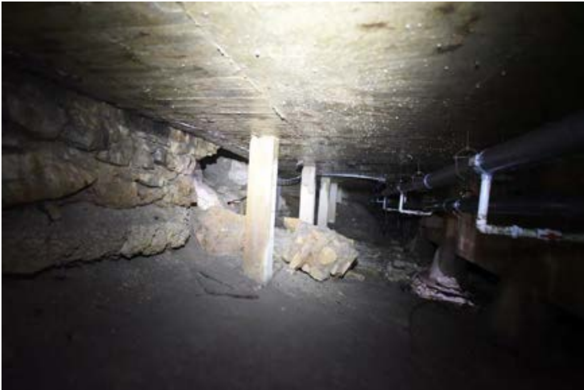
Figure 12. Same collapsed wall segment as in previous figure, looking opposite direction (northeast). Intact stone masonry wall is on the left with the undermined base visible.
