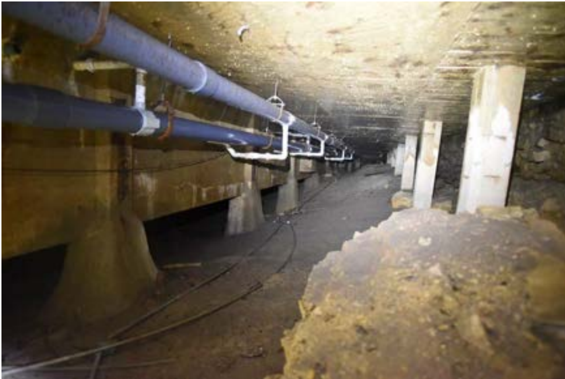
Figure 16. Looking southeast toward the Big Chief spring. Pool structure is on the left; collapsed stone masonry wall in the foreground; retained west side of the basin is on the right. Ahead in the distance, a large diameter concrete pipe is visible to the left of the columns; Big Chief spring is to the right of this.
