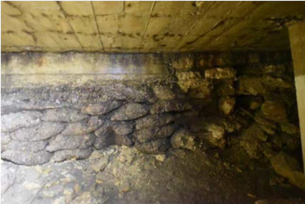
Figure 13. Wall repair using bagged materials.
