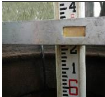
Recording measurement for manhole depth
