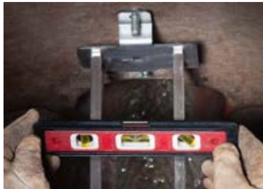
Confirm Level Side to Side
