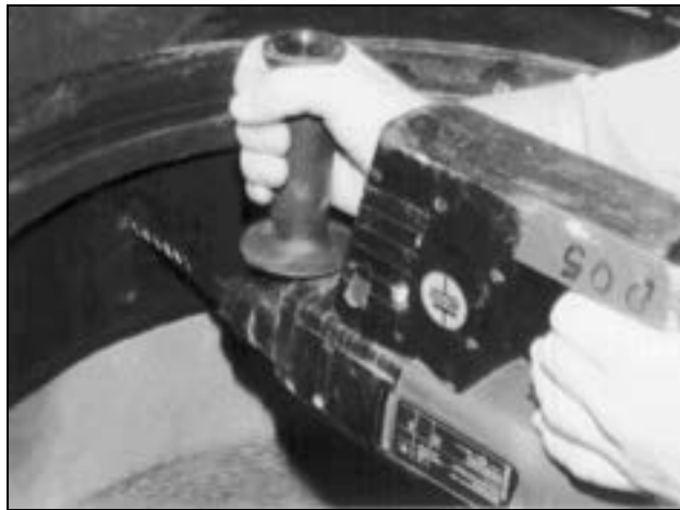
Drilling the hole in the manhole rim
