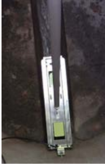
Run the Topside Extendable Retrieval Tool Down the Manhole
