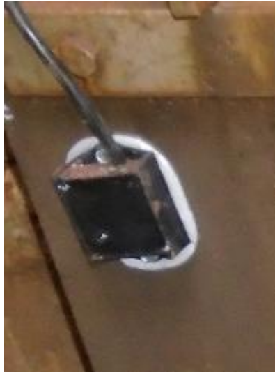
Inclinometer attached using Construction Adhesive
