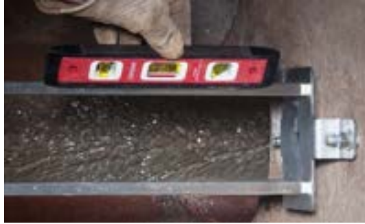
Confirm Level Front to Back
