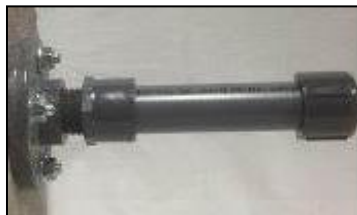
Screwing Wall Mount Bar into installed bracket
