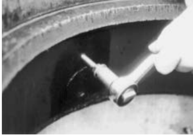
Installing the stud into the hole in the manhole rim
