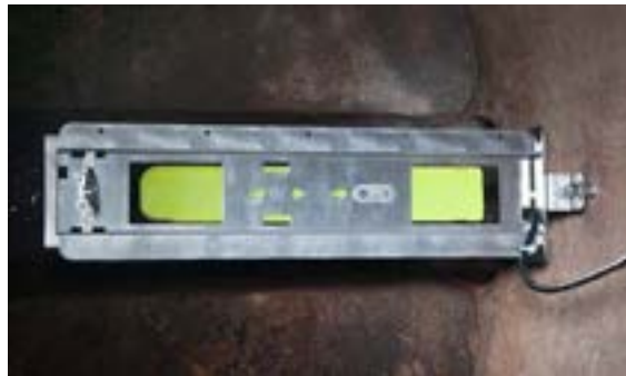
Installed Sensor Bracket on Wall Mount Bracket
