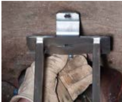
Place Lower Tab of Bracket on Lag Bolt and Finger-Tightening Bolt
