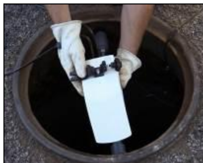
Unscrewing and opening shroud bracket
