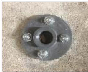
Securing bracket to the manhole wall
