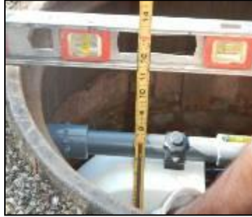
Recording physical offset at measurement intersection
