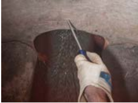
Mark Lower Tab Position for Mounting Bracket
