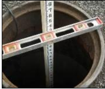
Placing Carpenter's level across open manhole frame
