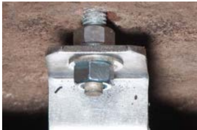
Stainless Steel Nuts and Washers Behind Mounting Bracket Tab for Leveling Purposes
