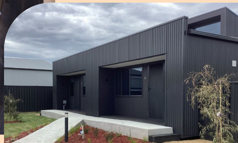
25 modular homes were built by Haven Home Safe in Horsham. Image: Haven Home Safe.
