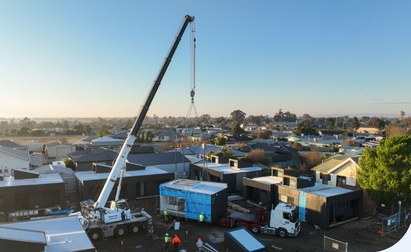
Craning a modular home into place at Haven Home Safe's new Horsham development. Image: Haven Home Safe.
