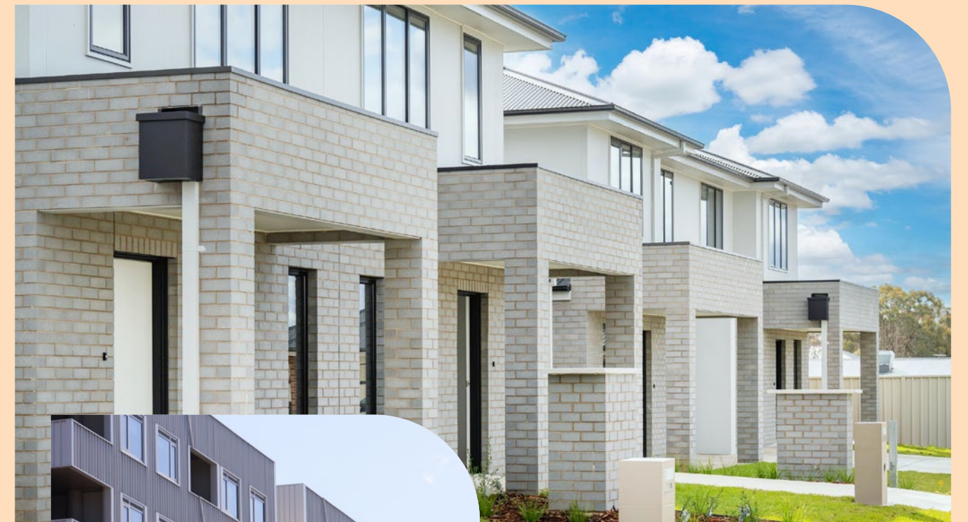
Six new homes for women were delivered by YWCA in Wodonga. Image: YWCA.
