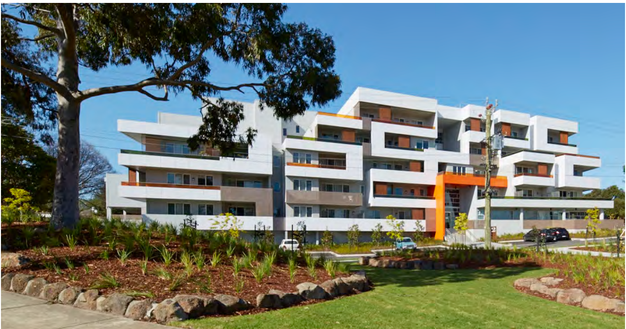
Ashwood Chadstone Gateway exterior
