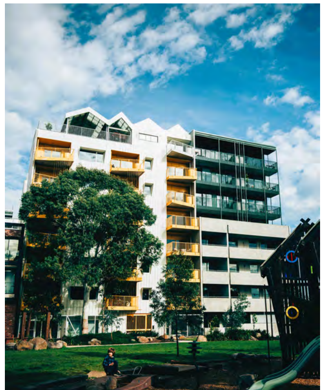
Nightingale Village – apartment exterior and nearby park.
