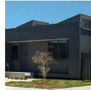
Haven Home Safe Modular Homes Horsham
