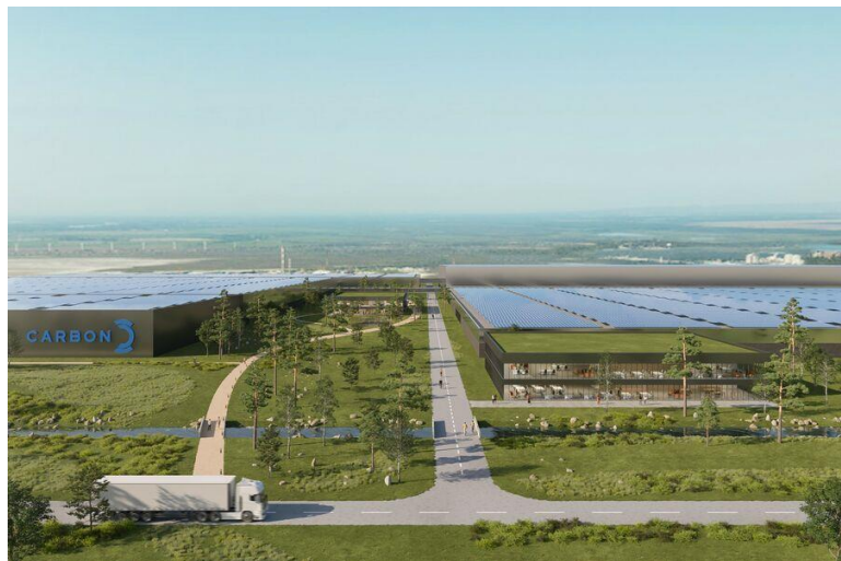
La future usine Carbon. ©Carbon
