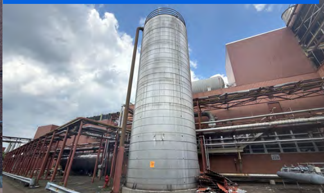
Fire Suppression & Chilled Water Tanks
