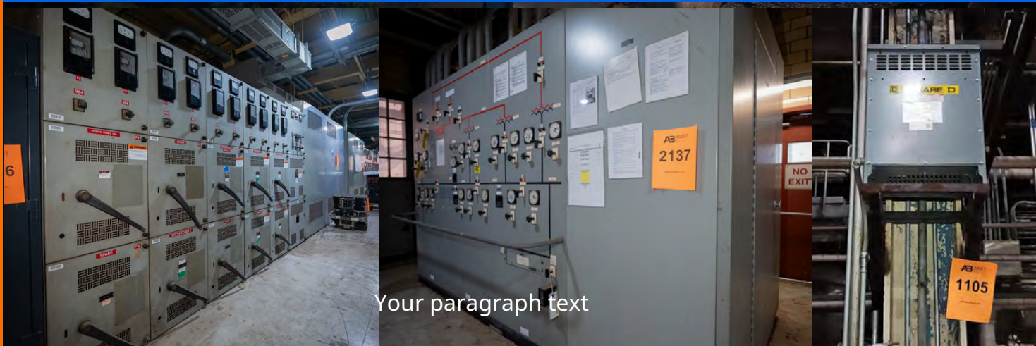
Substation-Class & Medium-Voltage Switchgears | Motor Control Centers (MCC)
