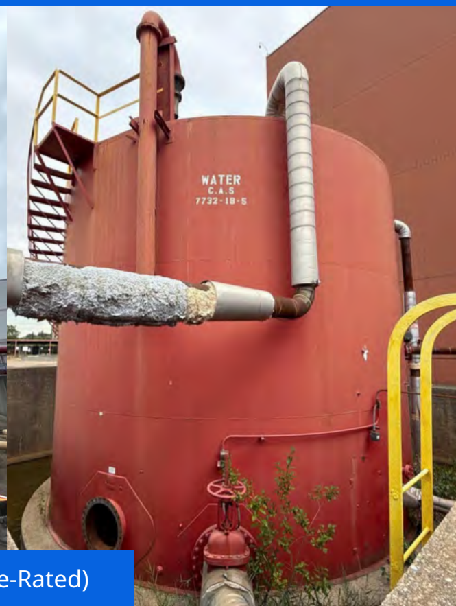
Fire Suppression & Chilled Water Tanks
