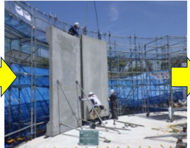
Installation of external walls
