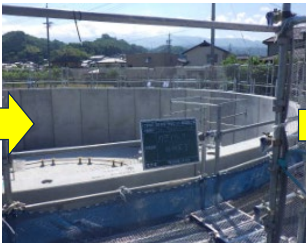
Installation of exterior walls completed
