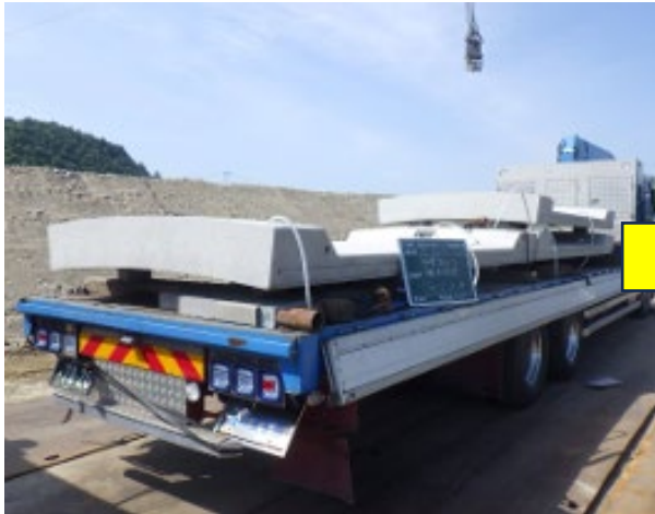
Carrying in the exterior walls
