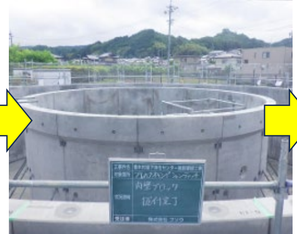
Installation of inner walls completed
