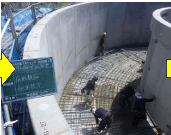
Bottom plate concrete works
