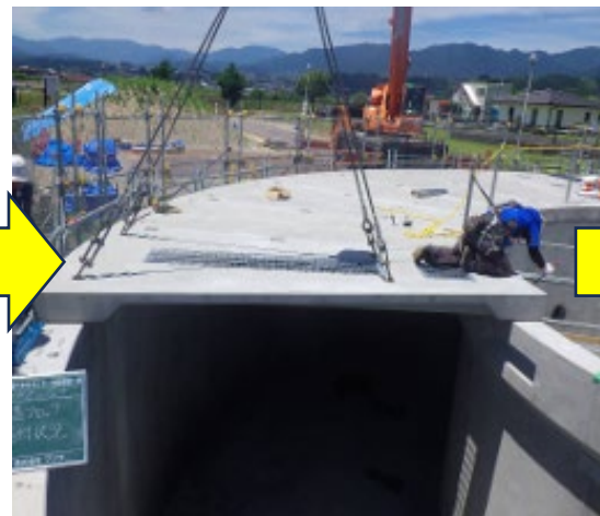
Installation of cover blocks
