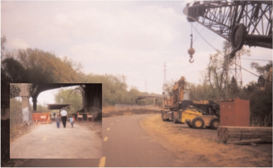
Construction equipment deployed in the trail corridor will be used to replace the decades-old bridge, which is in the background. Walkers (inset photo) go beneath the bridge.
