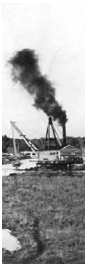
Equipment used to dredge the Chain of Lakes.
