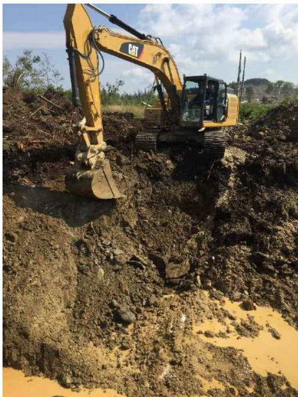
Plate 22. Trenching 2017 Raven Zone. Quartz briefly exposed in trench floor.
