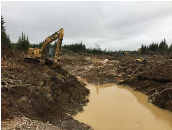
Plate 13. Elm Zone looking southwest, 2017 trenching program.
