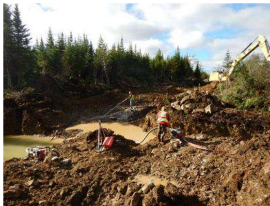
Plate 40. Trenching and washing Elm Zone 2017
