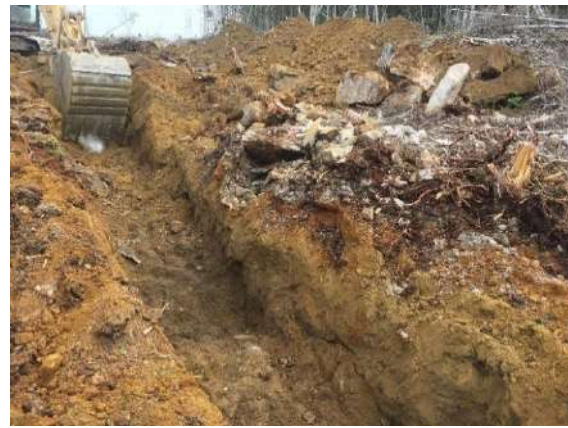
Plate 25. Trenching adjacent to frost-heaved quartz boulders, Red Ochre Complex.
