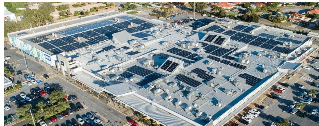
Solar Panels at Riverton Shopping Centre
