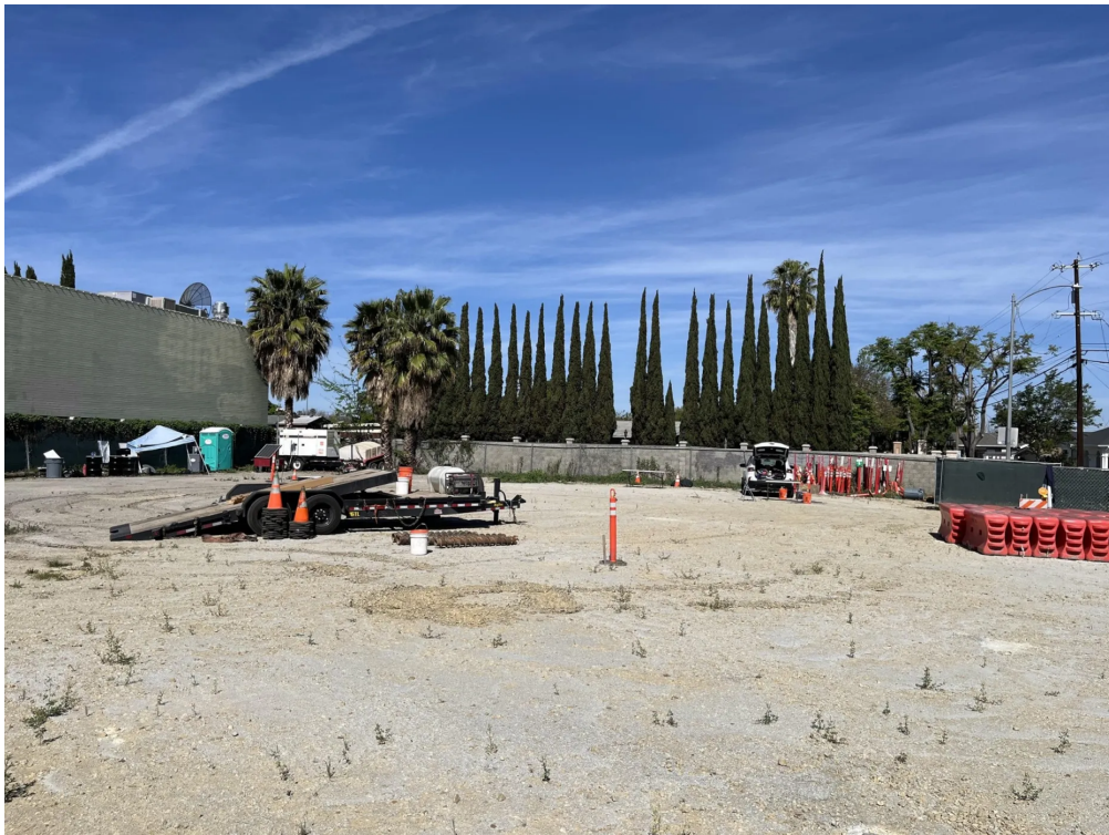
Housing development project site at 1135 East Santa Clara Street, as seen on March 26, 2026. (George Avalos/Bay Area News Group)
