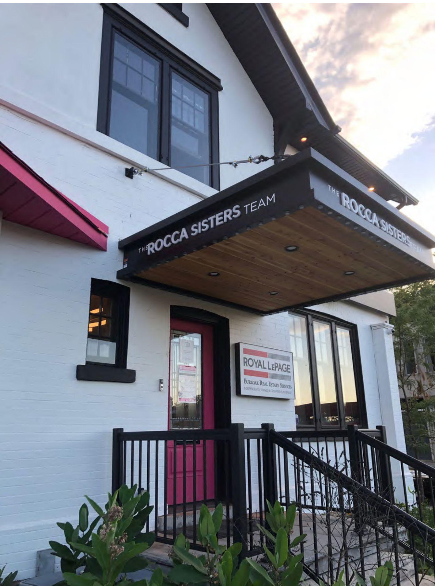
Highly Custom - Canopy Overhead
