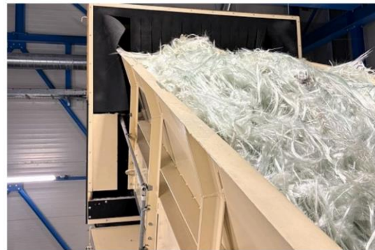
A portion of an industrial line at Owens Corning's L'Ardoise, France, facility, which is pioneering a circular glass recycling process. Source | Owens Corning
