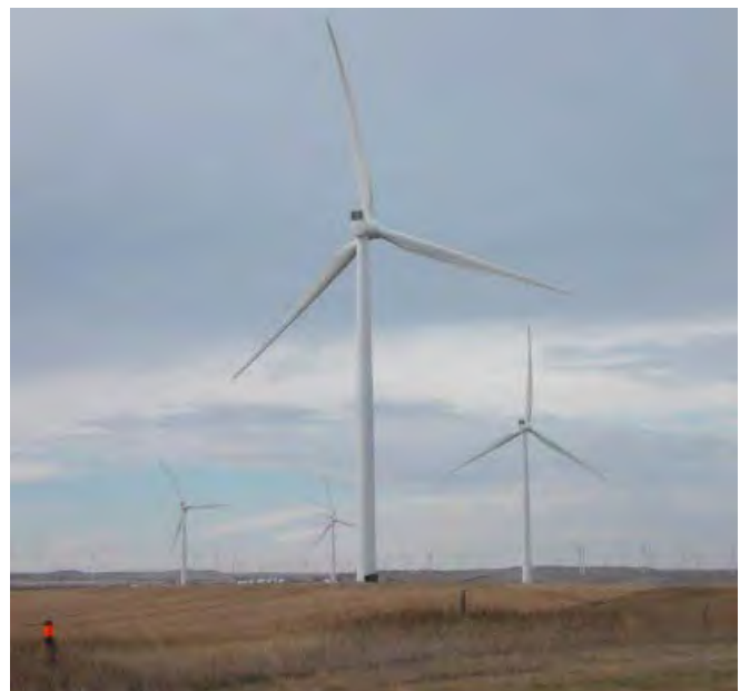
Figure 3.9: Example of a wind farm in North Dakota.
