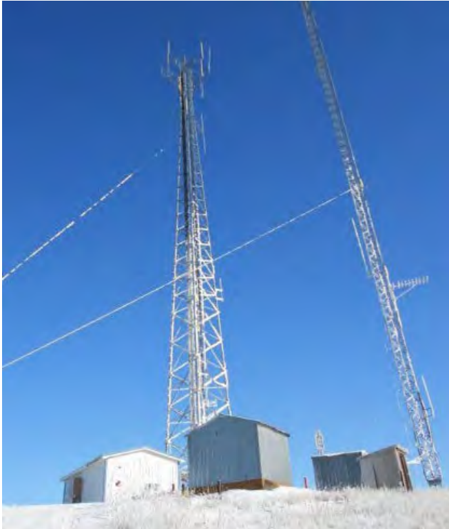
Figure 3.23: Example of vertical obstruction (communication tower).
