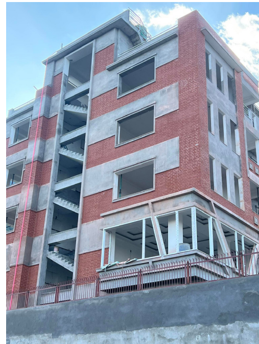
Safe House Under Construction
