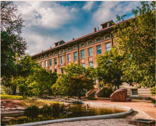
UT Austin's nineteenth school will gain a permanent home, thanks to a $100 million investment from the Board of Regents to renovate the Biological Laboratories building at Texas's flagship university.
