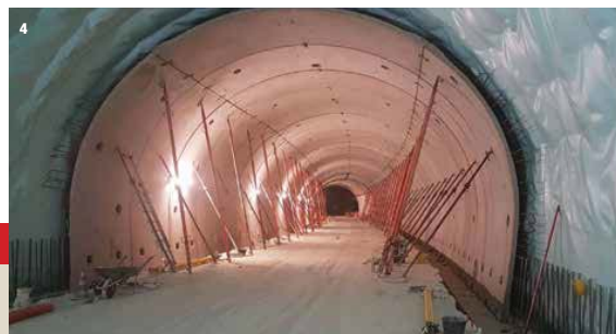
3. A1 motorway, South Florence, Antella tunnel: double slab retaining walls
