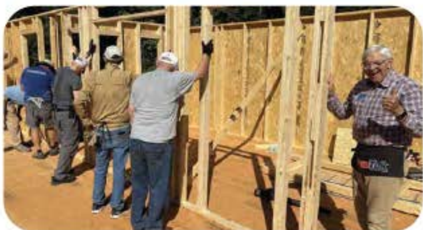
Residents volunteer with Habitat for Humanity to build the second home funded as part of the three-year commitment.
