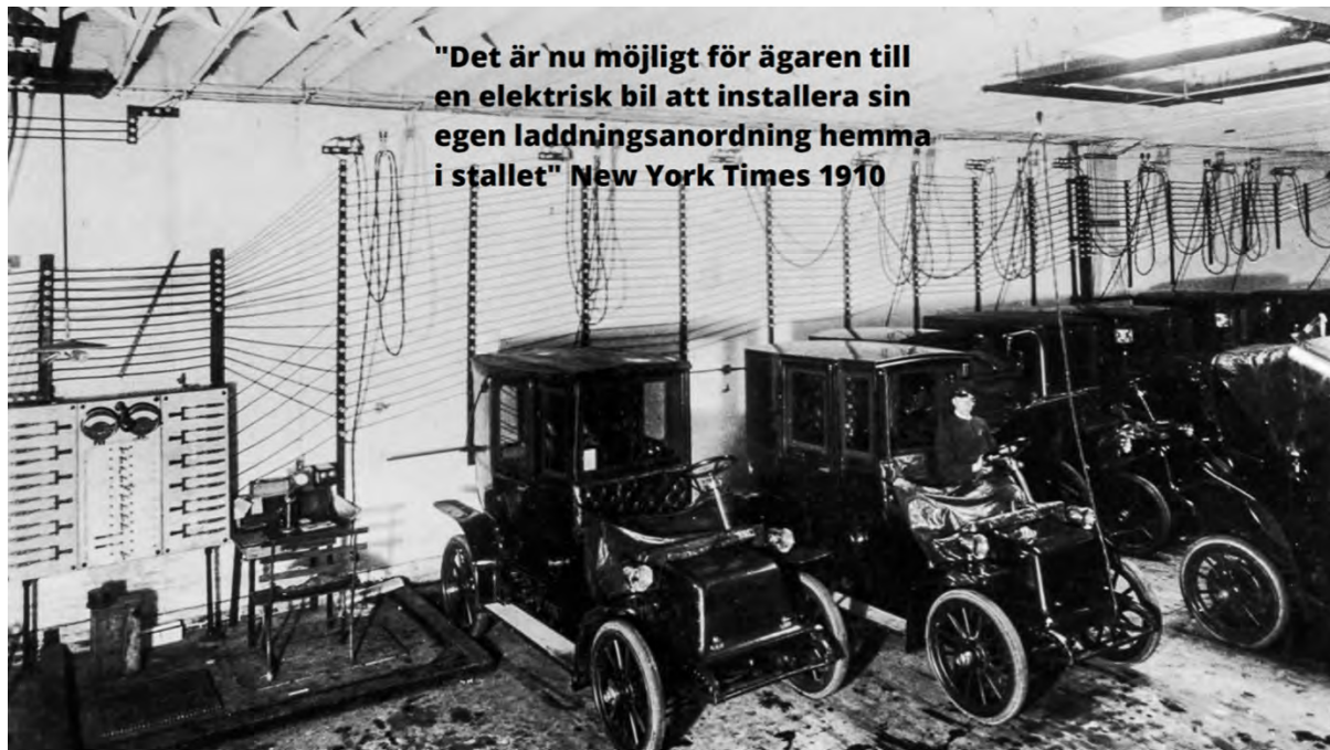
"It is now possible for the owner of an electric car to install his own charger at home in the stable" Source: New York Times, 1911, cited in Kilson (2016)
