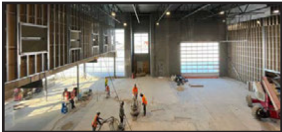
Indoor building progress in February 2025
