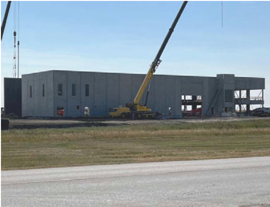
Building progress in August 2024
