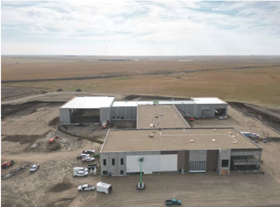
Building progress in October 2024
