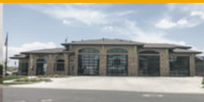
Station 2 9 Timber Ridge Pkwy. Severance
