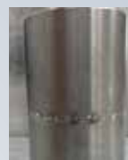
Pipe butt weld Ø 31.75 x 2 mm
