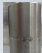
Pipe butt weld Ø 31.75 x 2 mm
