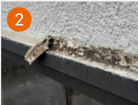
Failed Sealant
