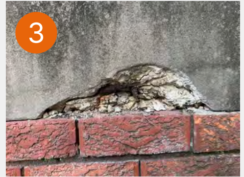
Concrete Deterioration
