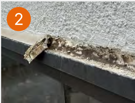
Failed Sealant
