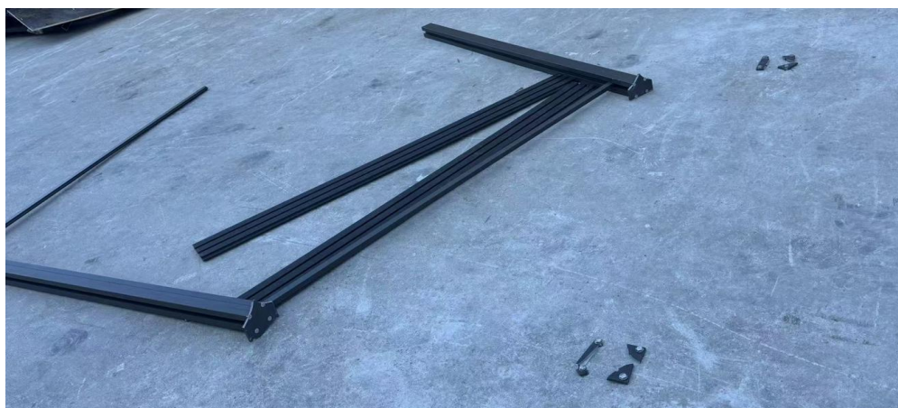
Photo 4. The fence specimen was damaged by the wind load at wind speed of 100 mph
