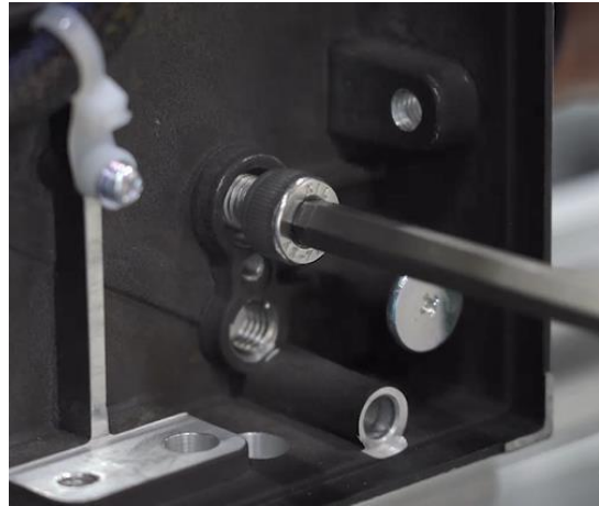
Fasten the Cabinet with the Hex Socket Head Screws M8*20 (Ensure that the Cabinet maintain horizontal and vertical during installation)
