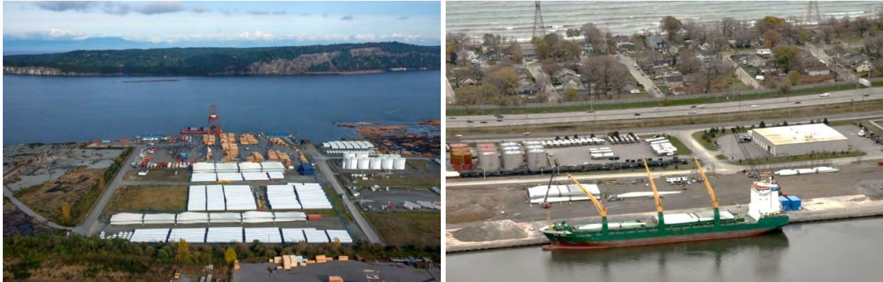
Figure 14: C.H. Robinson laydown yard (left) & vessel offloading to laydown yard (right)
