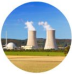
Nuclear Power Plant
