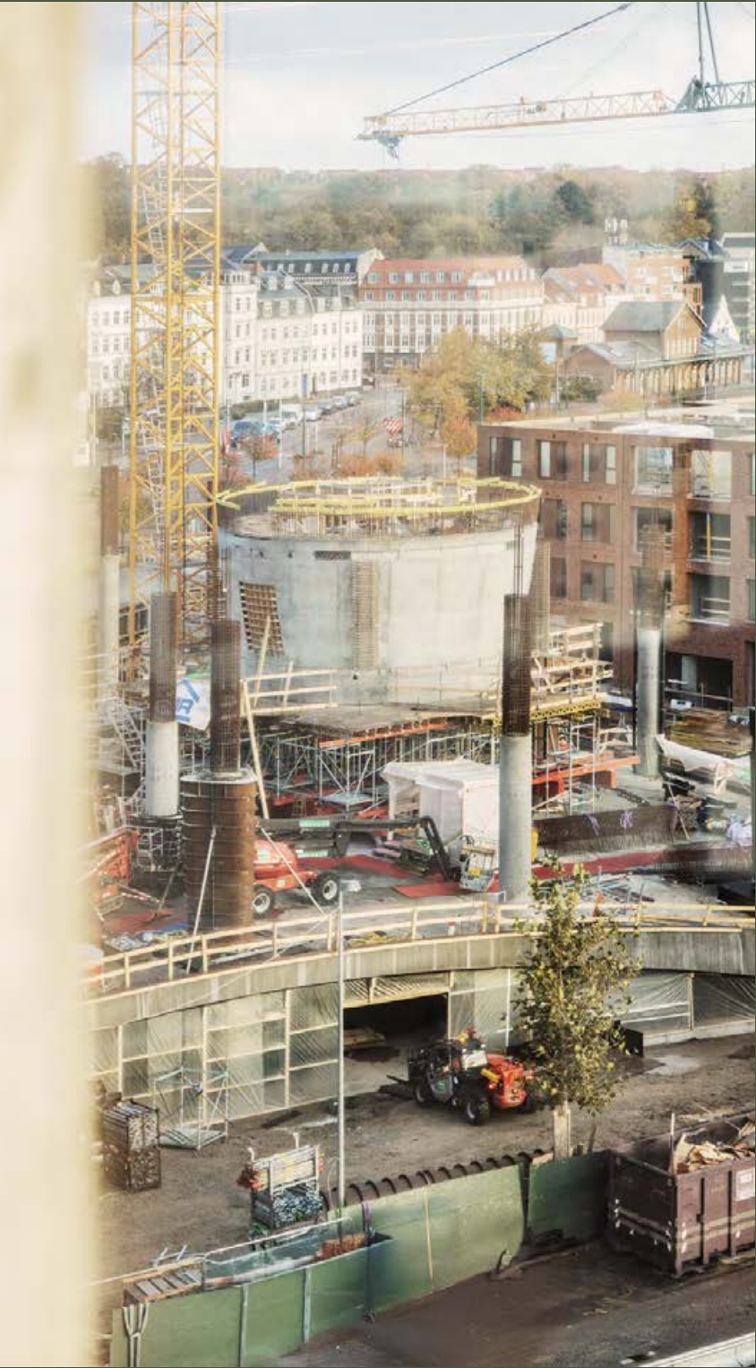
Hængslet The construction site for Hængslet - a new landmark on Aarhus Ø that will linking the island to the central Aarhus. The building, designed by Dorte Mandrup will host office spaces, and the ground floor will welcome visitors with a market hall, shops, and green public areas.
