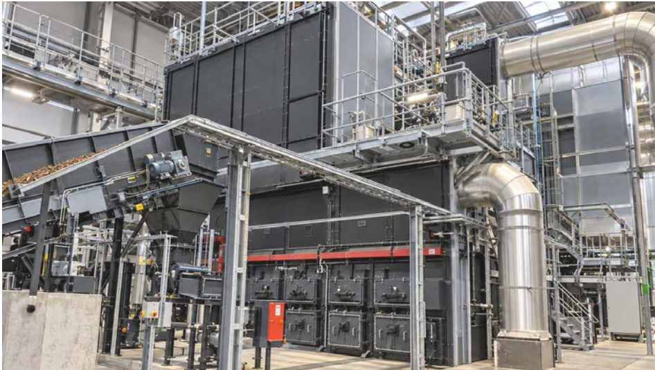
A Biomass Grate Combustion System
