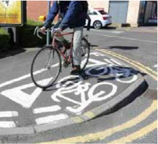
Nonsensical Miss-application of road-traffic design creates crazy results and damages respect.
