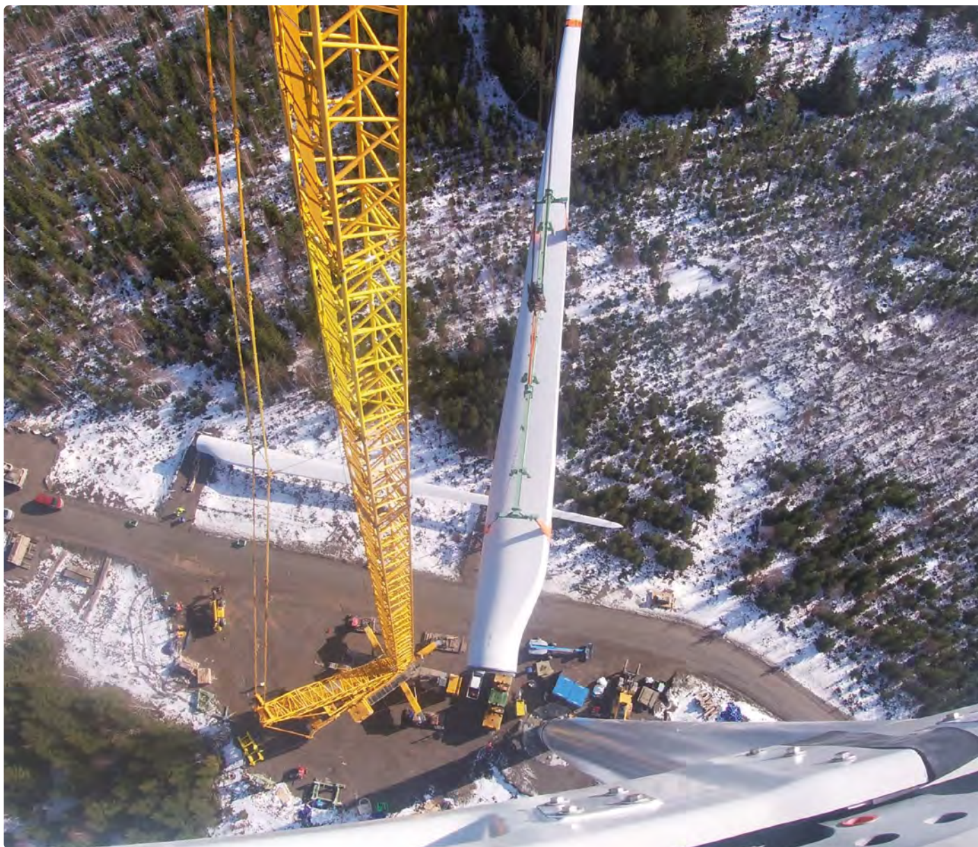
Ljungbyholm: Hoisting a blade into position
