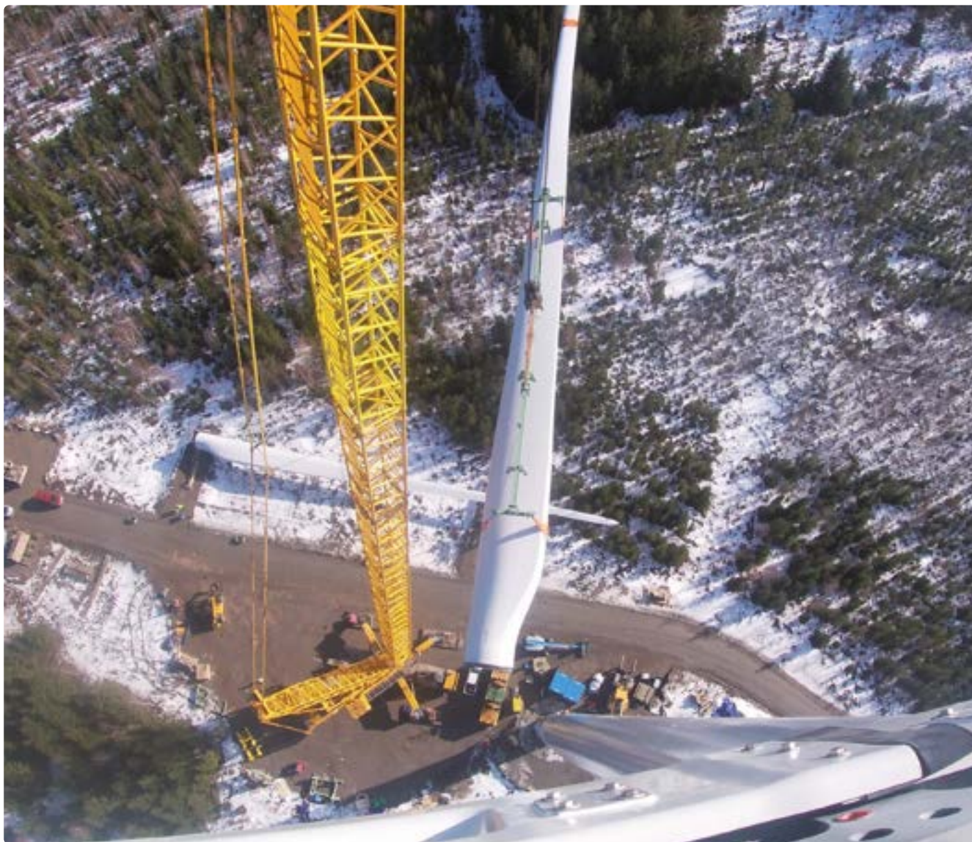
Ljungbyholm: Hoisting a blade into position
