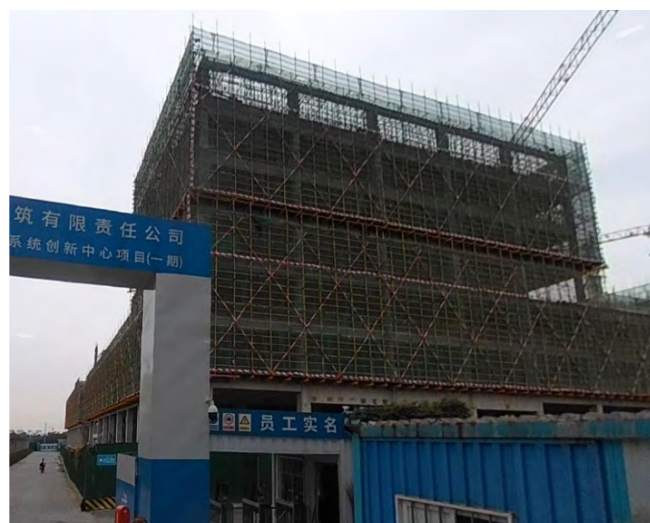
Figure 4: BOE (Chengdu) Smart Technology Innovation Center 58
