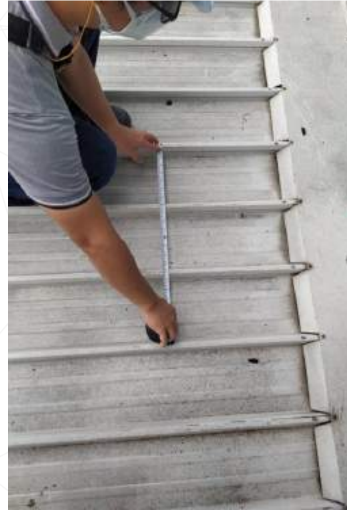
ROOF STRUCTURAL ASSESSMENT FOR PROPOSED ROOF MOUNTED SOLAR PV SYSTEM
