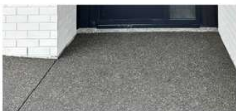
Exposed Aggregate concrete
