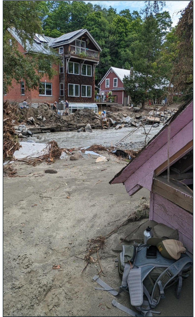
Riverbank damage to homes during the 2024 Plainfield flooding, where the water took not just the houses but the ground they stood on.
