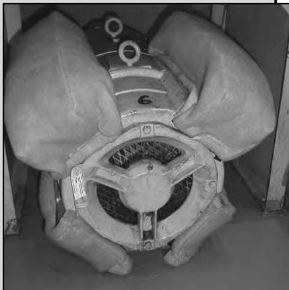
NEW CLEAN INSTALLATION (IMPERIAL 366)
