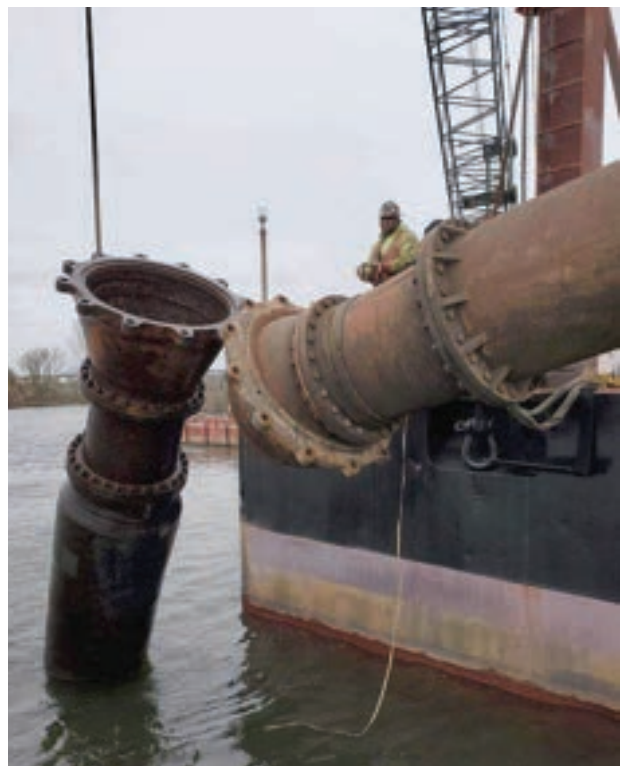
Members working under our contract with Philadelphia Ship Services recently reattached a 48" hose coupler for dredge spoils onboard a U.S. Army Corps of Engineers barge. Members working on that project included Kevin Barry, Chris Grupp, Brendan Joyce and Ryan Grupp.
