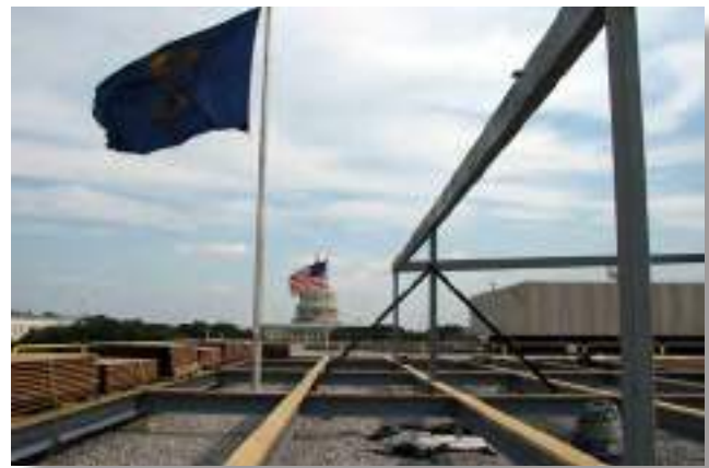
In late June, the construction workers get busy laying the support for the wood decking.
