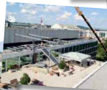
The steel lift took place on June 23. Throughout the course of the day all of the steel was set on the building along with 90 ipe panels. The steelworkers also assembled half of the staircase and the framing for the elevator and retractable awning that day.
