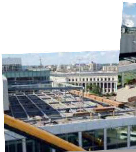
The steel lift took place on June 23. Throughout the course of the day all of the steel was set on the building along with 90 ipe panels. The steelworkers also assembled half of the staircase and the framing for the elevator and retractable awning that day.
