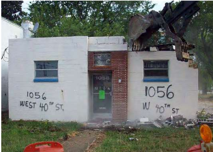
The old Norfolk Hall on 1058 W. 40th St. on the day it was demolished.
