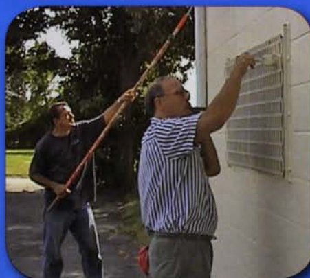
In Norfolk, Rep. Jeff Hauck organized a paint party to coat the exterior of our Union hall. Jeff got the job done dirt-cheap aided by a terrific band of members who volunteered their time and hard work to help make a huge improvement at the hall. Constantine Cristescu is at left with Jeff Hauck in action with paint brush and cell phone (dispatching a job?).
