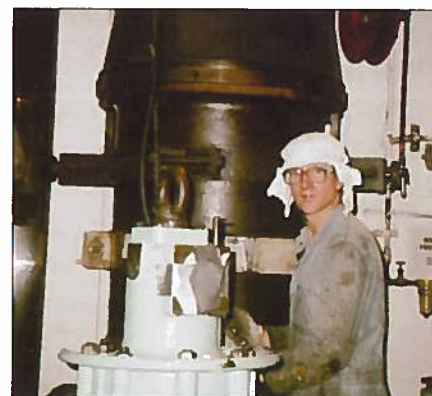
Brian Collins, 1st A/E on the CSX KODIAK, working the crane after removing liner and piston.
