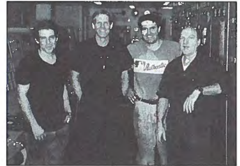
In the SEALAND PRIDE 's control room are MEBA members (l-r) Bryant Salvesen (3rd A/E), Scott Manchester (1st A/E), James R. Nolan (2nd A/E) and Duane Dennis, Chief Engineer.
