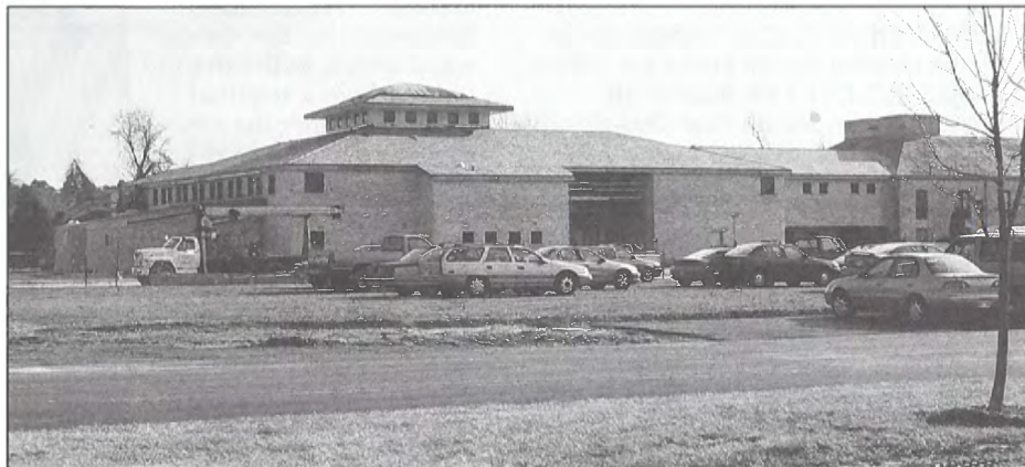
The exterior work has been completed on the new Luebke Center at the School. The excitement begins to crescendo for the grand opening this Spring.
