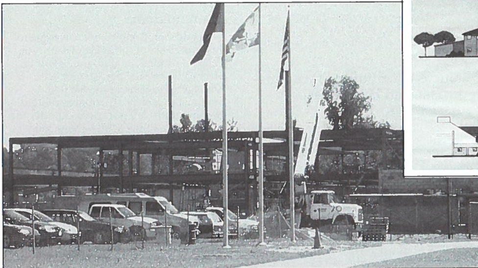
This eyesore will transform into a fully-functional multi-purpose facility by June.
