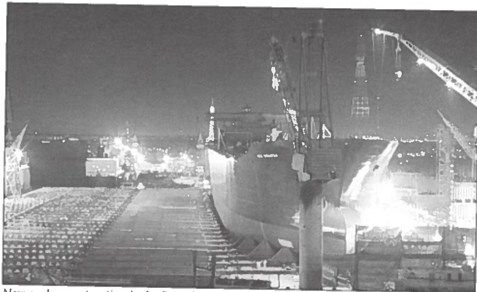
Now under construction is the first of at least three ARCO Millennium Class tankers. MEBA engineers will operate the most modern and most environmentally friendly crude oil tankers in the world fleet under the recent agreement between the union and Alaska Tanker Co.
